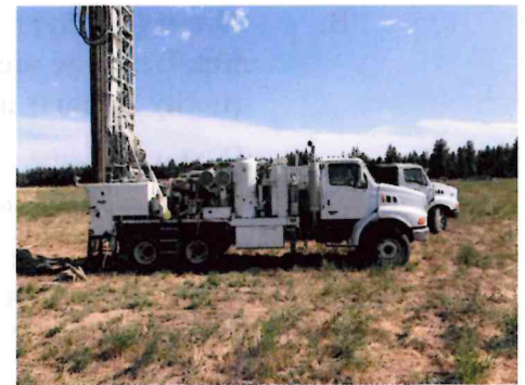
Typical truck-mounted RC rig
